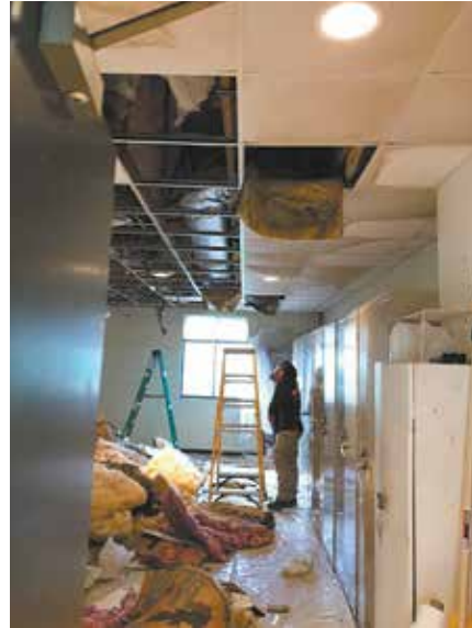
Wet insulation is taken down
